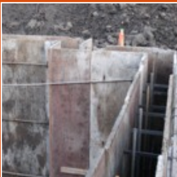
Top: The timbers in place Bottom: The concrete forms before pouring
